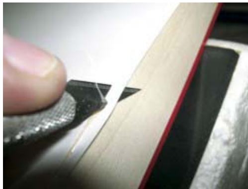
Raise covering away from center rib using sharp #11 blade to cut away overlap that prevents a strong adhesive joint.
