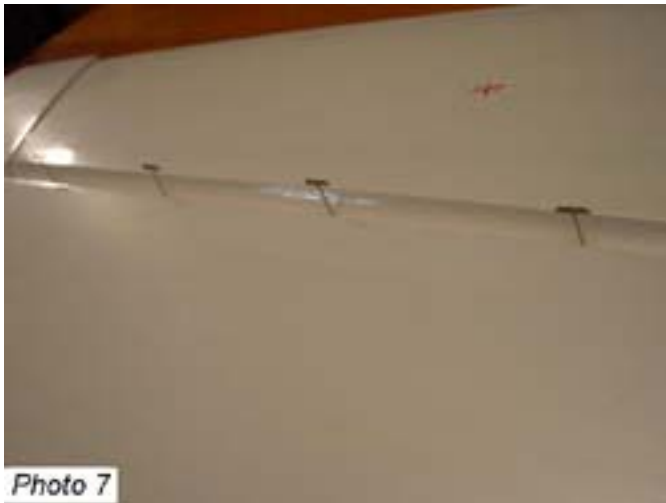
PHOTO 7 - Positioning all hinges prior to gluing
